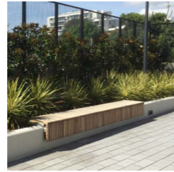
Concrete bench with timber battens
