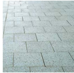
Concrete unit paving
